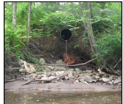
Figure 4. A Stormwater Outfall Discharging Untreated Runoff to a Stream (Photo: FB Environmental)
