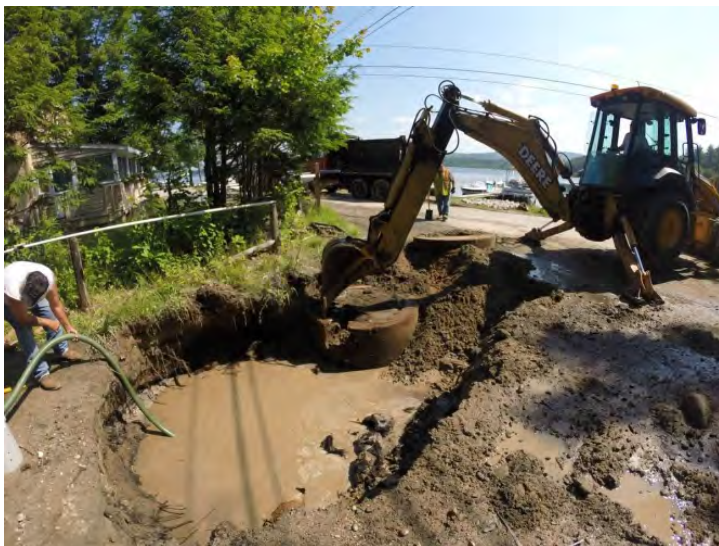
Pre-existing structure – note highly compacted sediment
