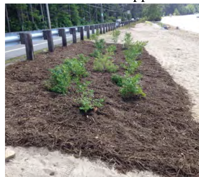
Figure 12: Rt 153 beach after buffer & erosion control mulch YCC installation
