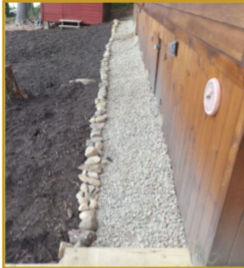
Dripline Trench - Traps roof runoff and directs it into the ground. An alternative to gutters.
