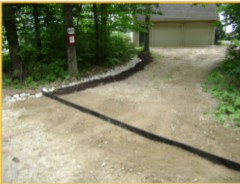
Rubber Razor - strips of hard rubber are partially buried in the driveway, placed on an angle to divert stormwater into an adjacent trench or natural area.
