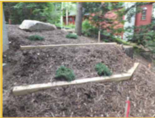
Water Bars - 6"x6" lumber is installed on a slope with crushed stone on the uphill side to trap and divert stormwater. Water bars are left slightly raised to slow water down and can be used as seen above, or placed in a pathway in shorter lengths to function as steps.
