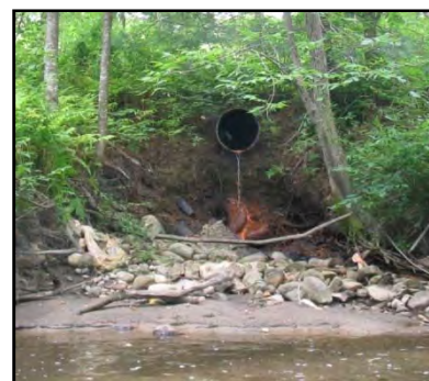
Figure 4. A Stormwater Outfall Discharging Untreated Runoff to a Stream (Photo: FB Environmental)
