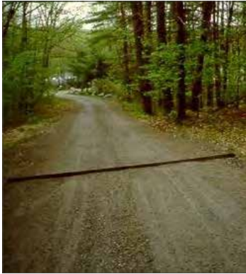
Rubber Razors —Direct water off the driveway and into vegetation with rubber razors.
