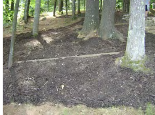
Ortiz Waterbar and Erosion Control Mix After
