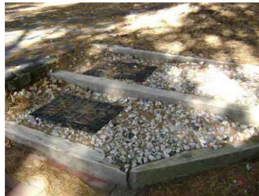
Darling Retrofit Infiltration Steps After
