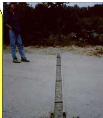
Open Top Culverts —Direct water off the driveway with open top culverts.
