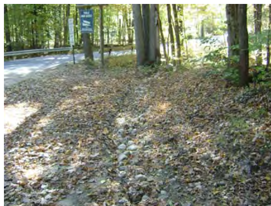
Robinson Road Infiltration Trench After
