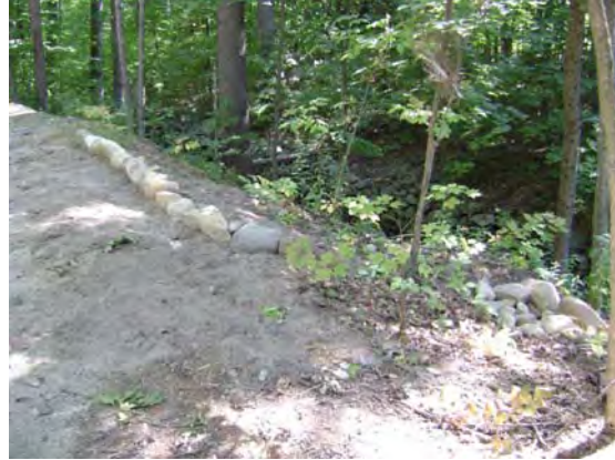
Canal Road Waterbar and Drywell After
