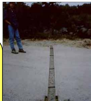
Open Top Culverts —Direct water off the driveway with open top culverts.
