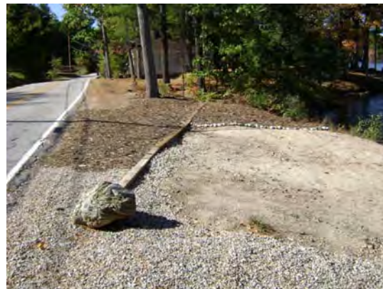
Golden Waterbar and Erosion Control Mix After
