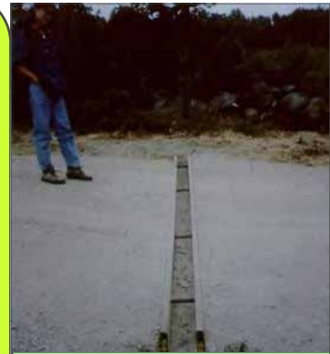
Open Top Culverts —Direct water off the driveway with open top culverts.
