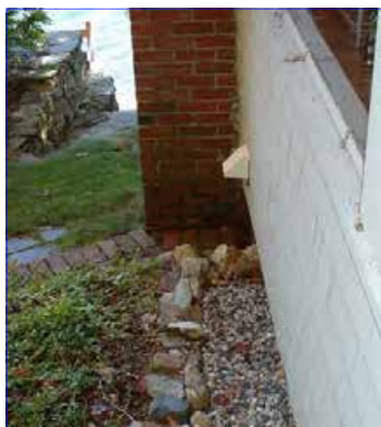
Roof Runoff —Install stone-filled trenches along roof drip-line to help infiltrate runoff.
