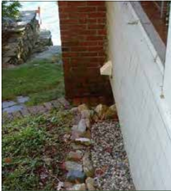
Roof Runoff —Install stone-filled trenches along the roof dripline to help infiltrate runoff.
