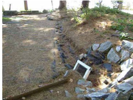
Binette Drywell and Trench with Filters
