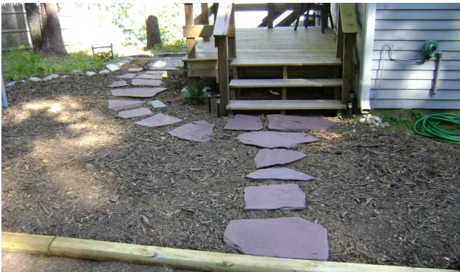
AWWA YCC Project on Lake Ivanhoe—Erosion Control Mulch (ECM) with slate walkway.
