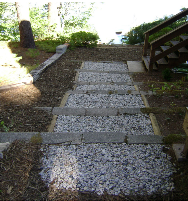
AWWA YCC Project on Lake Ivanhoe - Infiltration Steps
